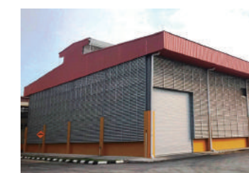
Drying facility designed to direct sunlight to the drying area
